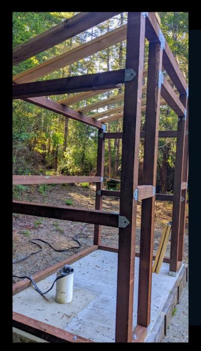
In the fall of 2022, concrete was poured, and framing completed for secure enclosures to house the mini treatment plant and wellhead.
