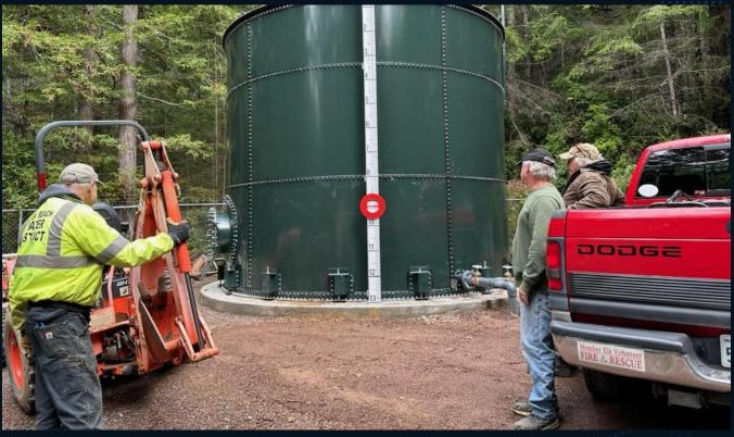
Construction of Tank 5, plumbing and electrical connections between Tank 5, Well 5, and Tank 4 were completed in early December.
