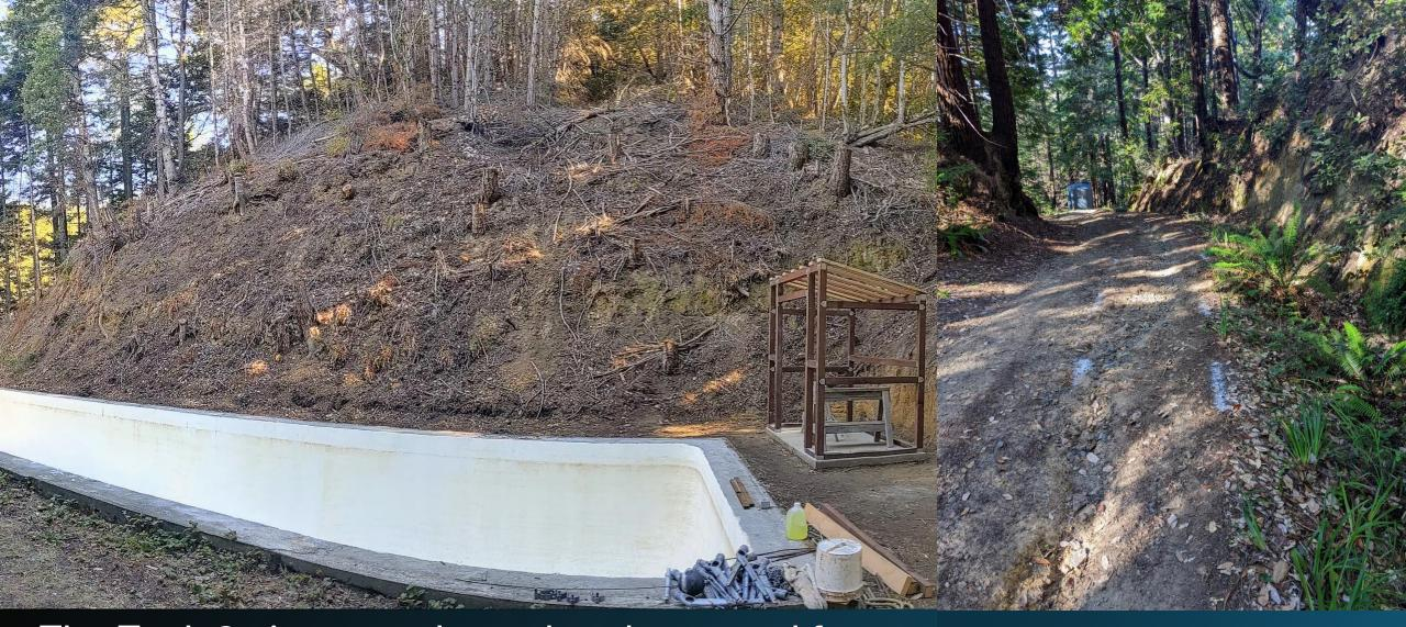
The Tank 2 site was cleared and prepped for delivery of the new cover and the roadway was marked for trenching.
