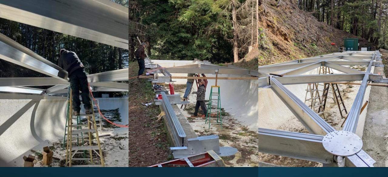
The Operations crew installed the girders for the new Tank 2 cover.
